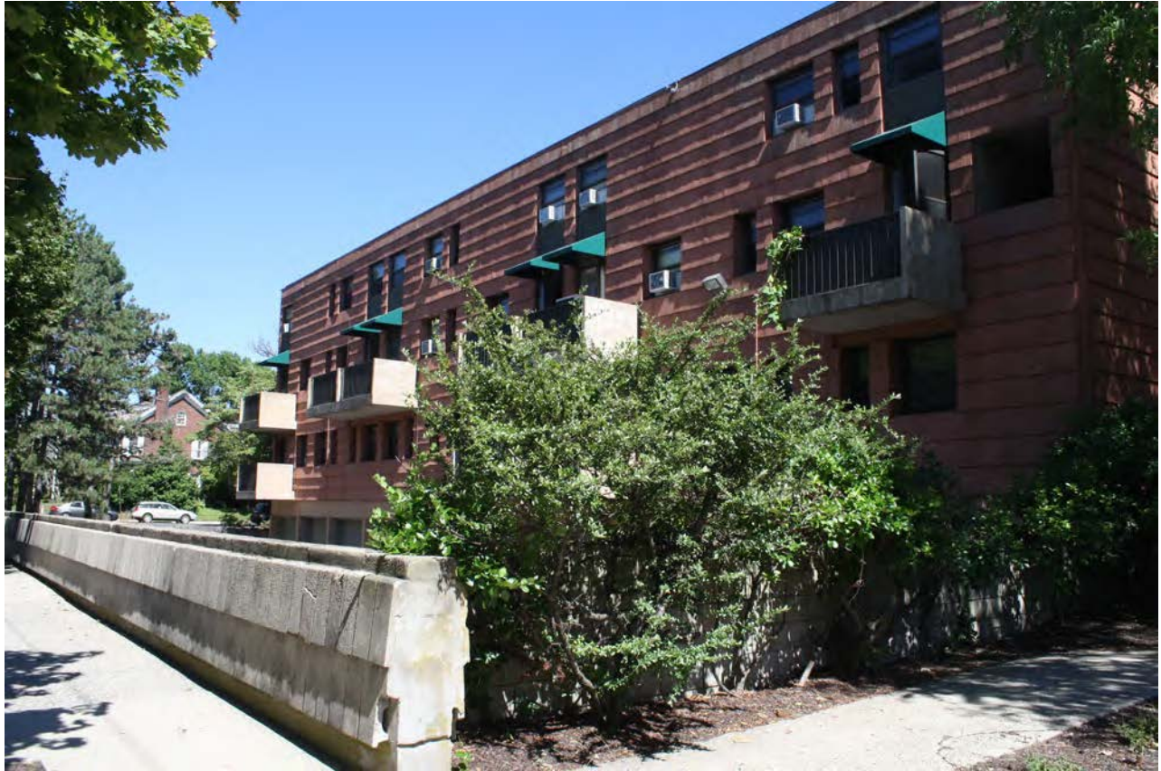
Photo 7. West elevation view of the Dwight Street side of Trade Union Plaza, camera facing north. The perimeter wall consists of the same custom block masonry as the building walls.
