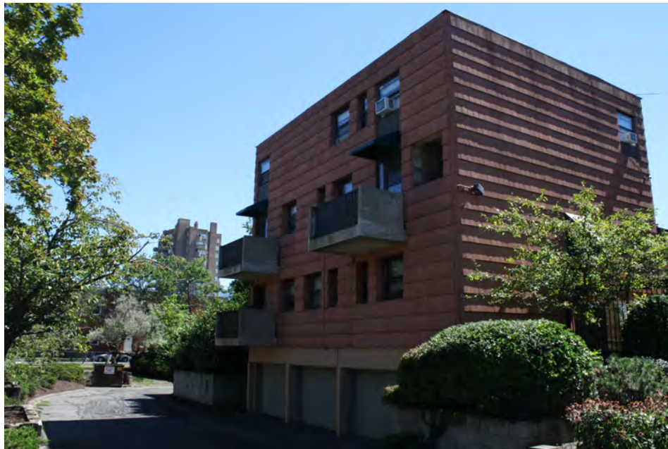
Photo 4. North elevation view of the George Street side of Trade Union Plaza, camera facing east. In the distance at rear is the 1965 Crawford Manor senior housing tower designed by Paul Rudolph.
