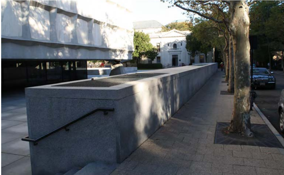
Figure 17. Detail view of landscape feature along Wall Street. The wall incorporates mechanical ventilation intakes; camera facing east. Note that the street grade slopes gently down toward the east, with the sidewalk meeting the plaza elevation at the area west of Woodbridge Hall.
