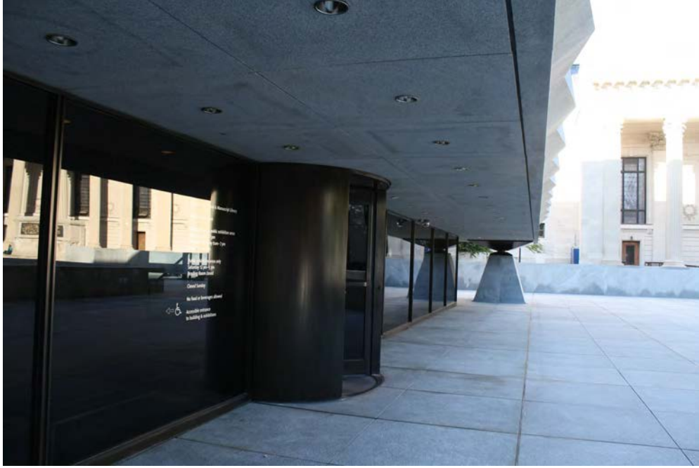
Figure 10. Exterior detail view of east side and entry facing toward Commons; camera facing north.
