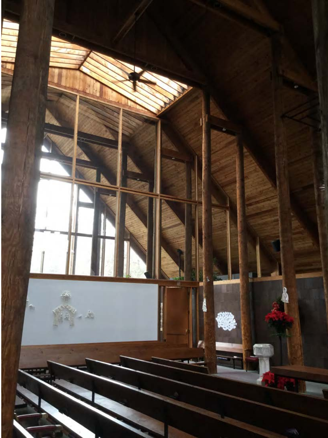
Photo 11. Interior view of the sanctuary, camera facing northwest, showing the skylights and glass partition between the Copeland Room to the west, and the sanctuary.
