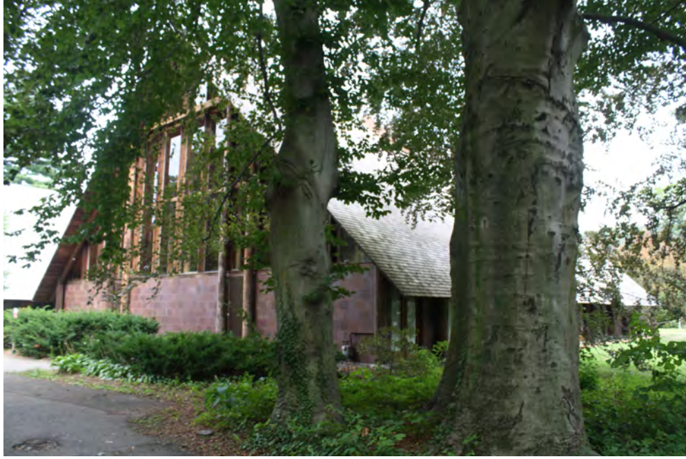
Photo 8. Southwest view from the rear driveway, camera facing northeast.
