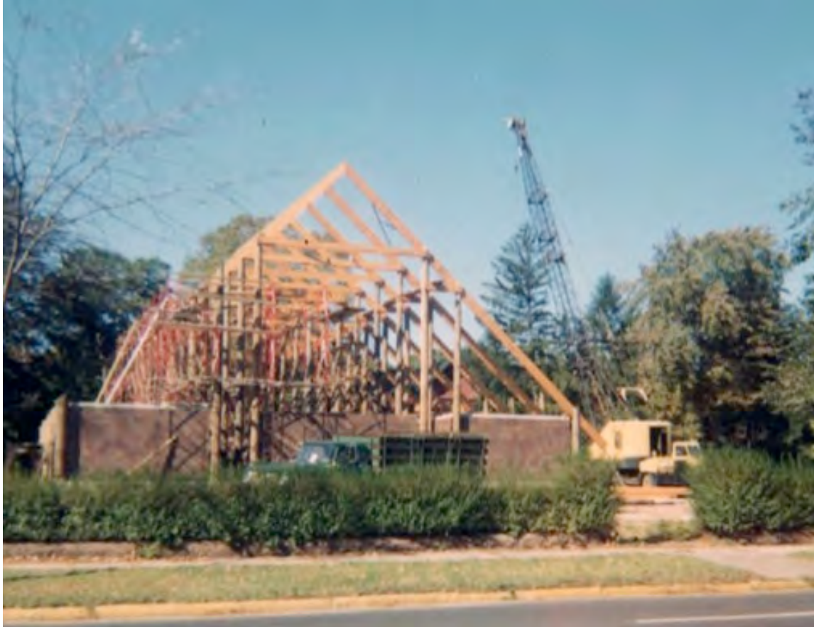
Photo 20. Photograph during construction, camera facing west. Photo courtesy of Jim Owens.
