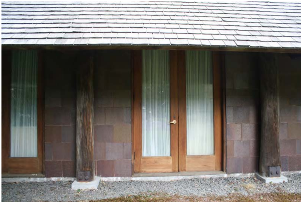
Photo 6. Detail view of south elevation, camera facing north.
