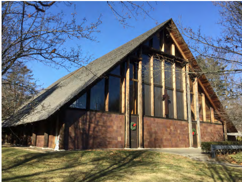
Photo 4. Southeast view, camera facing northwest. Note the original signage at right.
