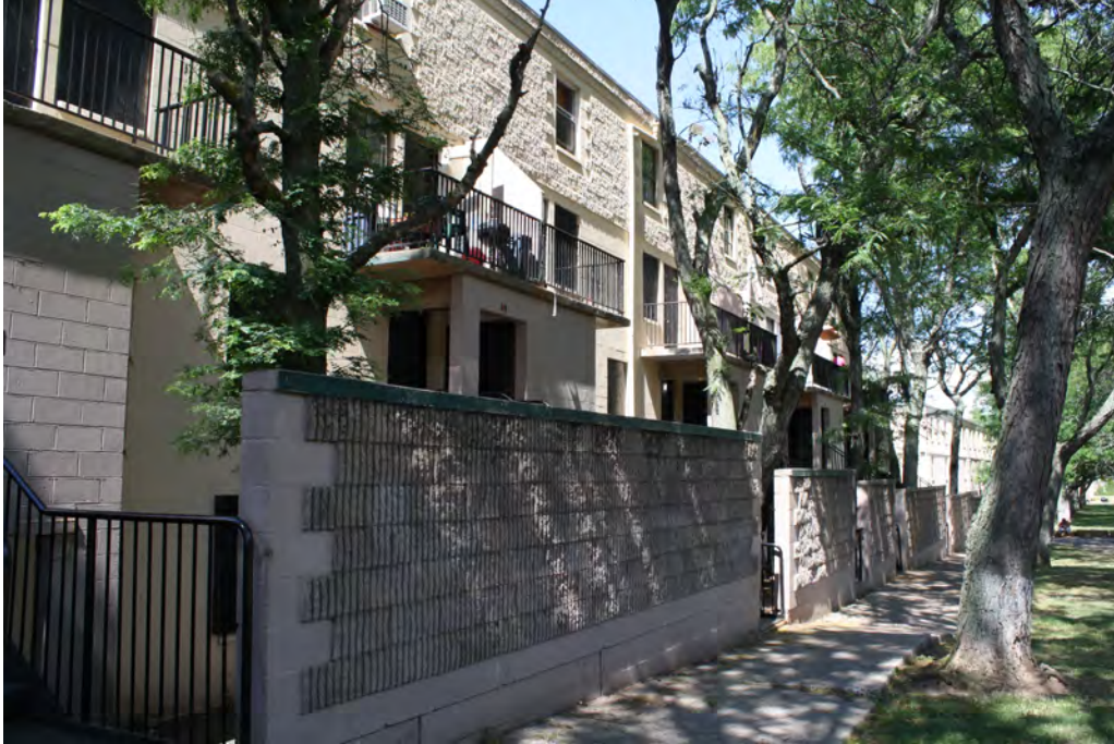
Photo 9. Southwest view of the Columbus Avenue building south elevation; camera facing east.
