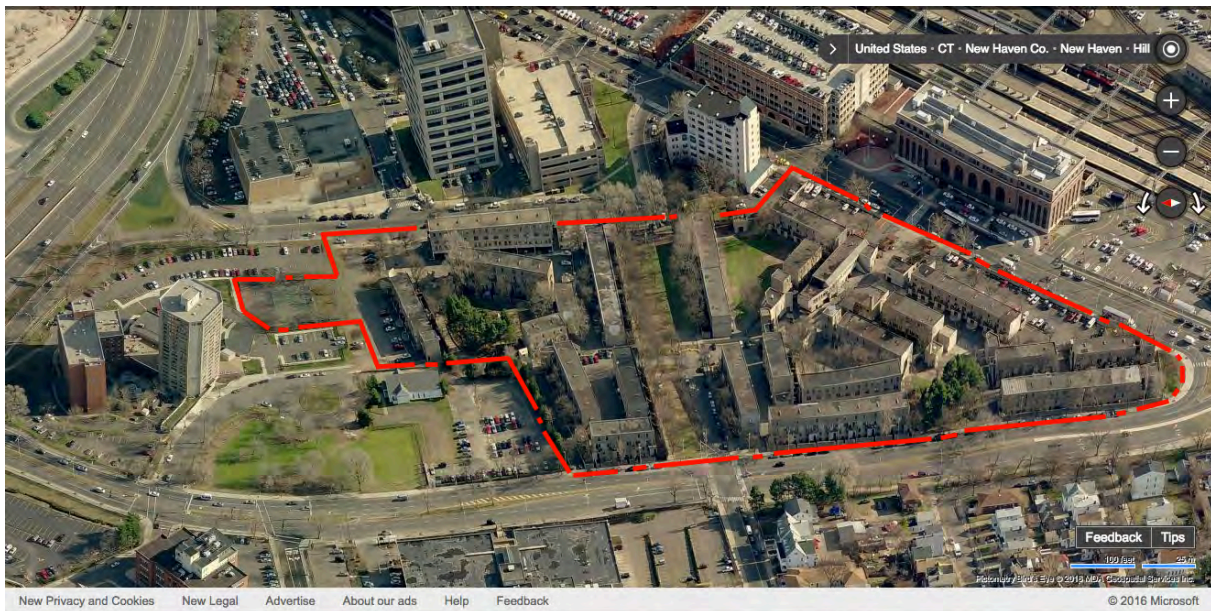
Figure 2. West aerial view of Church Street South. Base image from Bing Maps accessed 11/17/2016. Annotated to show the extent of the development site.
