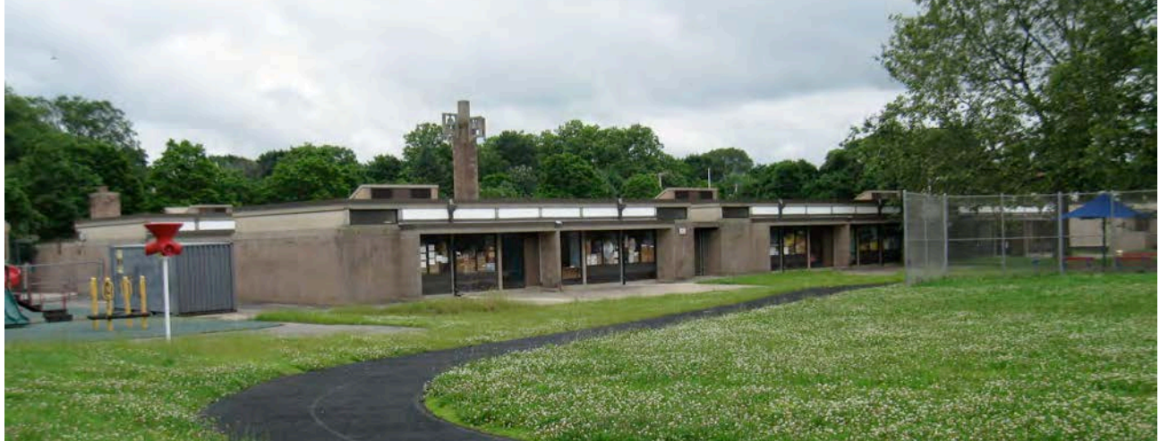
Photo 7. Northeast view, camera facing west. The paved area outside the classroom windows indicates the original courtyard extent. Clerestory windows have been fill in with white panels.
