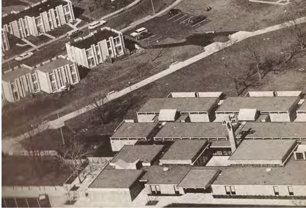
Figure 3. West aerial view of Helene Grant School and Florence Virtue Homes in early 1960s, camera facing northeast (Metz, 24). Note the classrooms with private walled outdoor courts, the clerestory windows between the structural roof girders, and the open court containing the bell tower.
