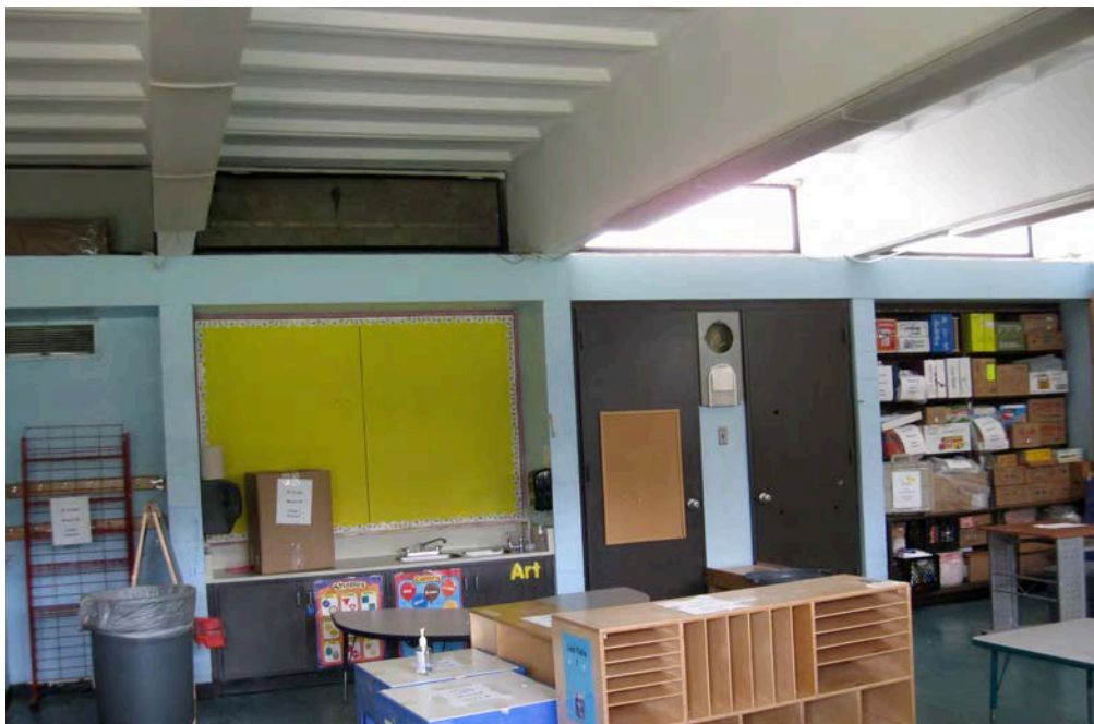
Photo 10. Interior view of typical classroom south wall; camera facing south.
