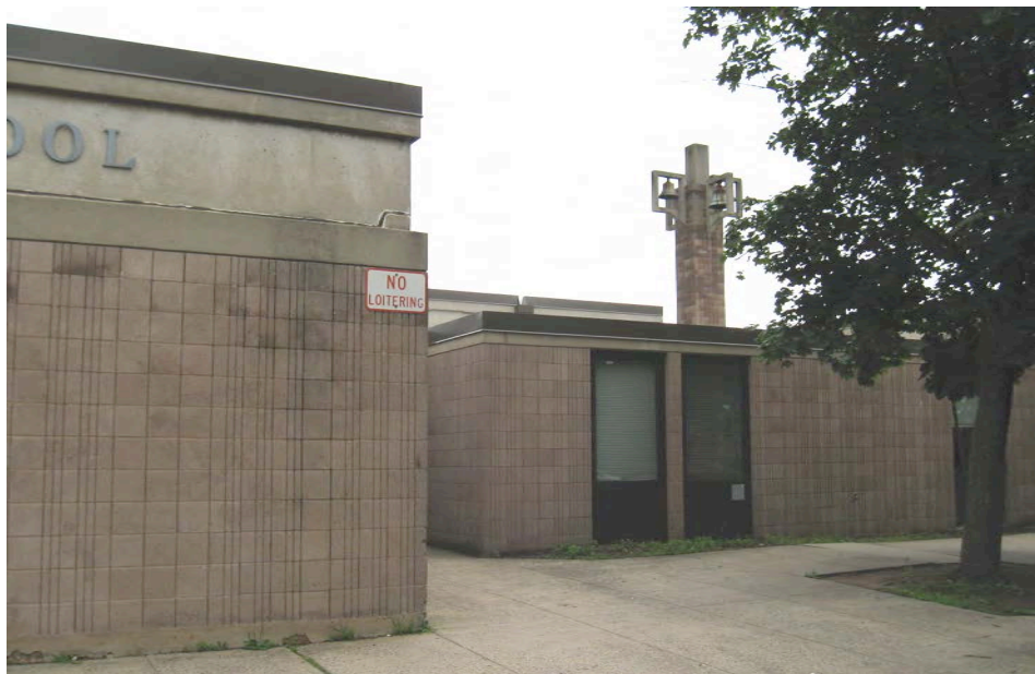
Photo 6. Southeast view showing the bell tower; camera facing northwest.
