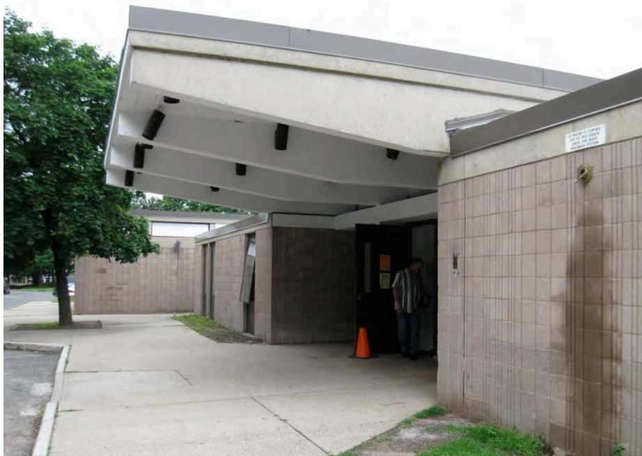
Photo 5. Southwest view of the entrance with its cantilevered canopy; camera facing north. Note the exterior wall material consisting of scored concrete masonry. The upper frieze of smooth concrete forms a unifying course around the building, with blocks of higher roofline with clerestory windows above the frieze, as visible at the left rear.
