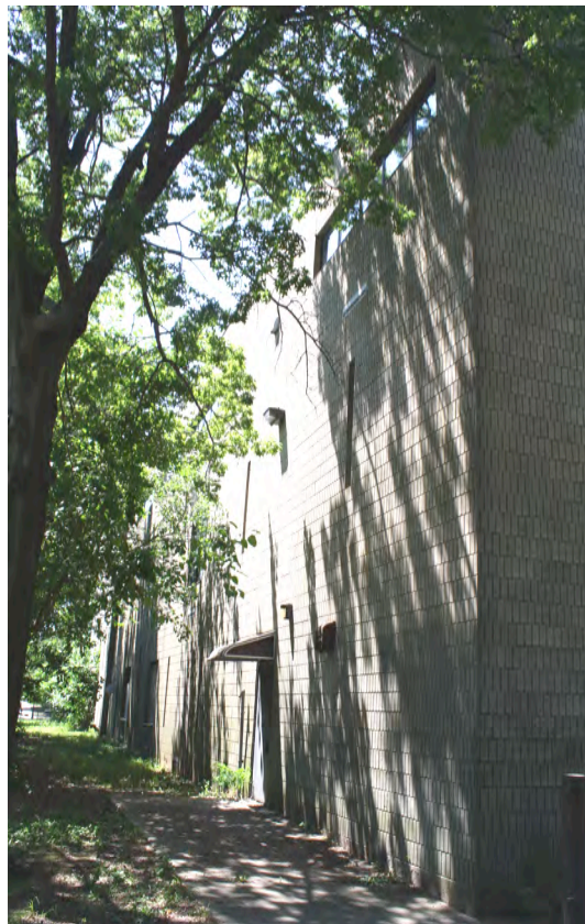
Photo 6. East view; camera facing southwest.
