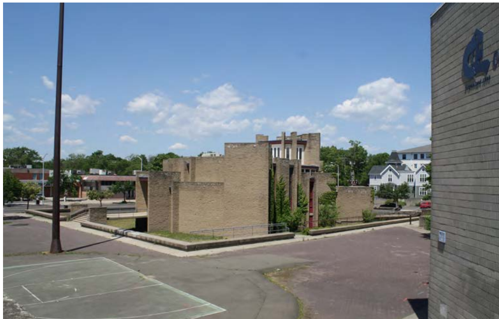
Photo 9. View west from upper plaza; camera facing northwest toward the Dixwell Congregational Church and Dixwell Plaza shopping.
