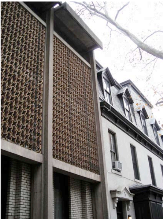
2. Detail, pierced block screen & concrete frame.
