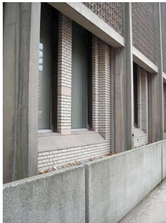
3. Detail, original brick and cast-stone façade.
