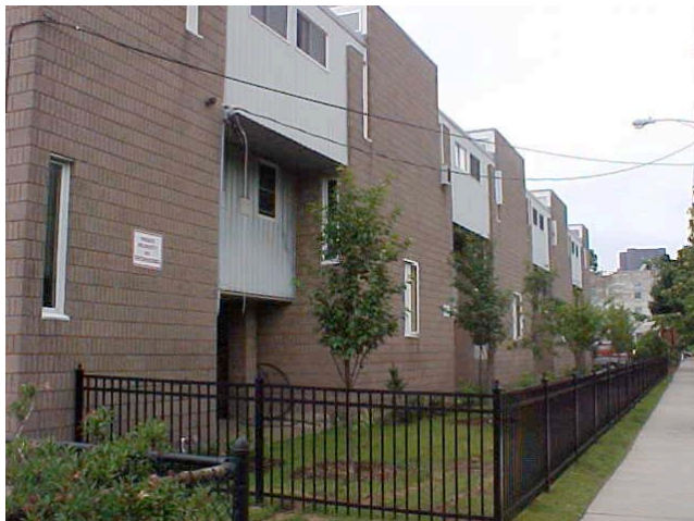
10. Wooster Street (north) elevation – New Haven Assessor's photograph, before painting, mid-2000s.
