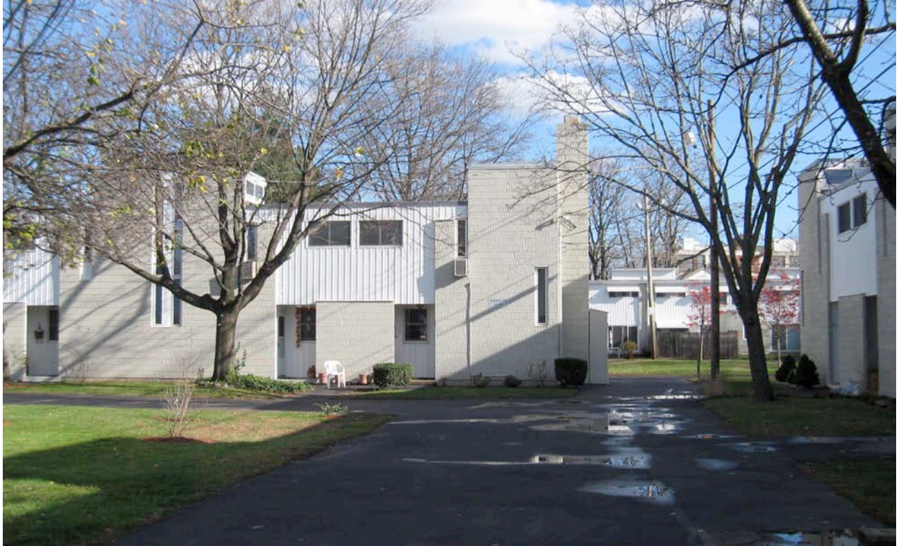
16. Front (west) elevation of typical two-story building facing interior quadrangle, camera facing east.
