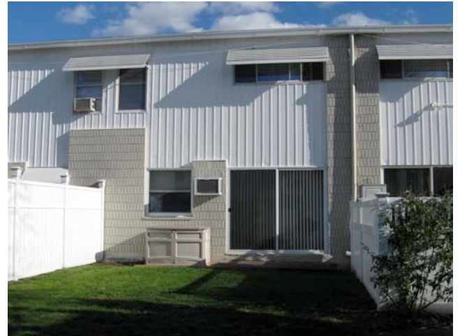
15. Typical rear building elevation, 2009.
