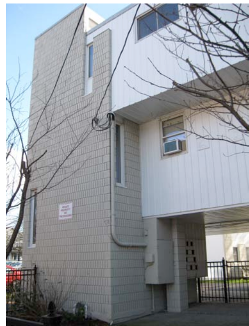
11. Wooster Street (north) elevation detail, after painting, December 2009.
