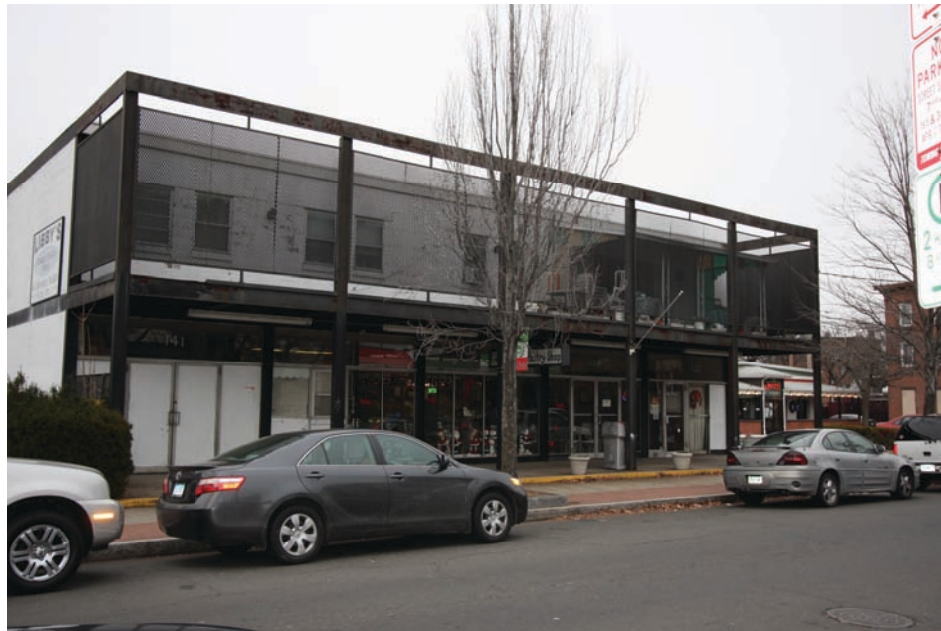
1. Southwest view from street, camera facing northeast.
