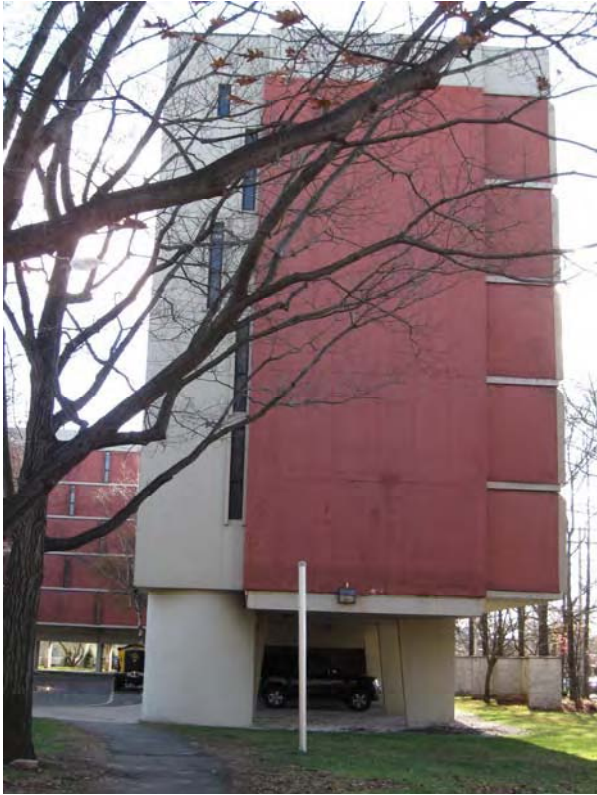
3. North view, camera facing south.
