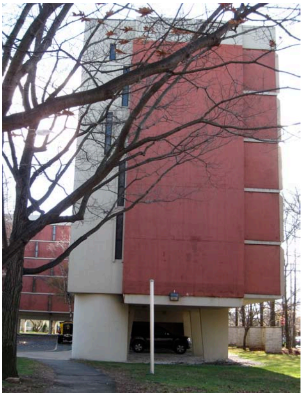
3. North view, camera facing south.
