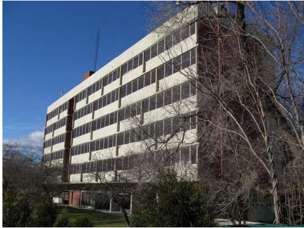
1. Southeast view of south building from Warren Street, camera facing northwest.
