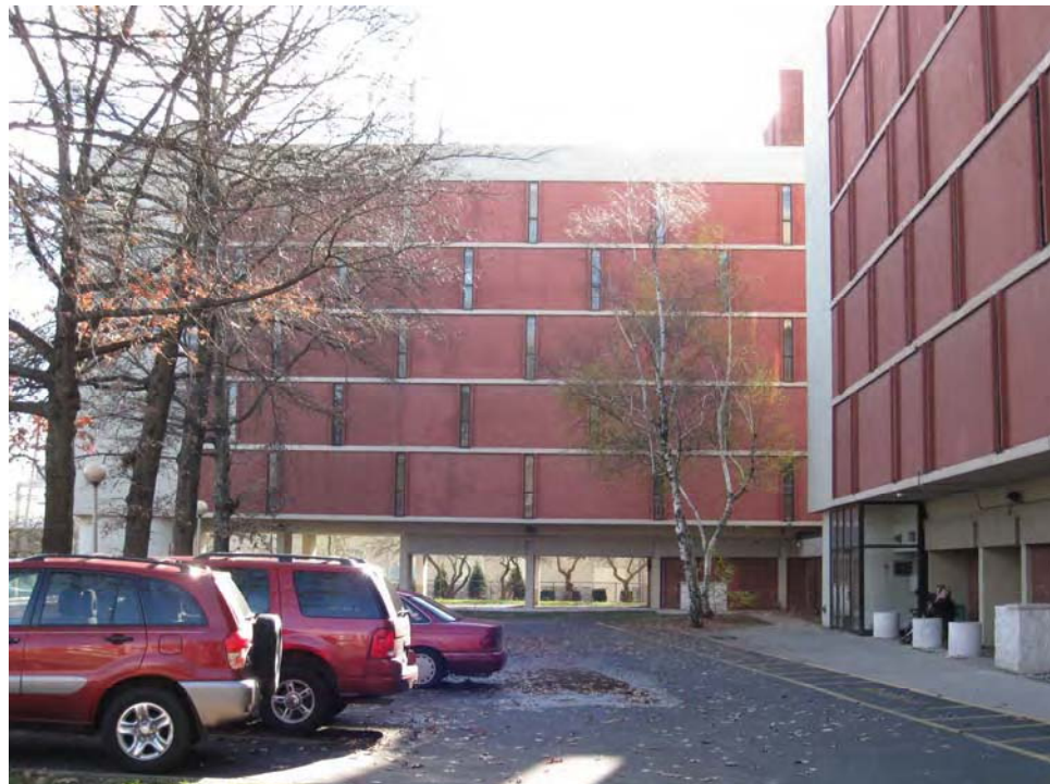
2. North view from parking, camera facing south; south building in distance, west building at right.
