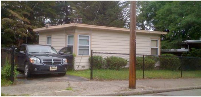
2. 3 Hilltop Road, camera facing south.
