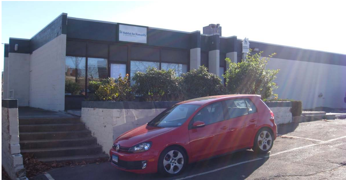
1. West view from Fair Street, camera facing east.
