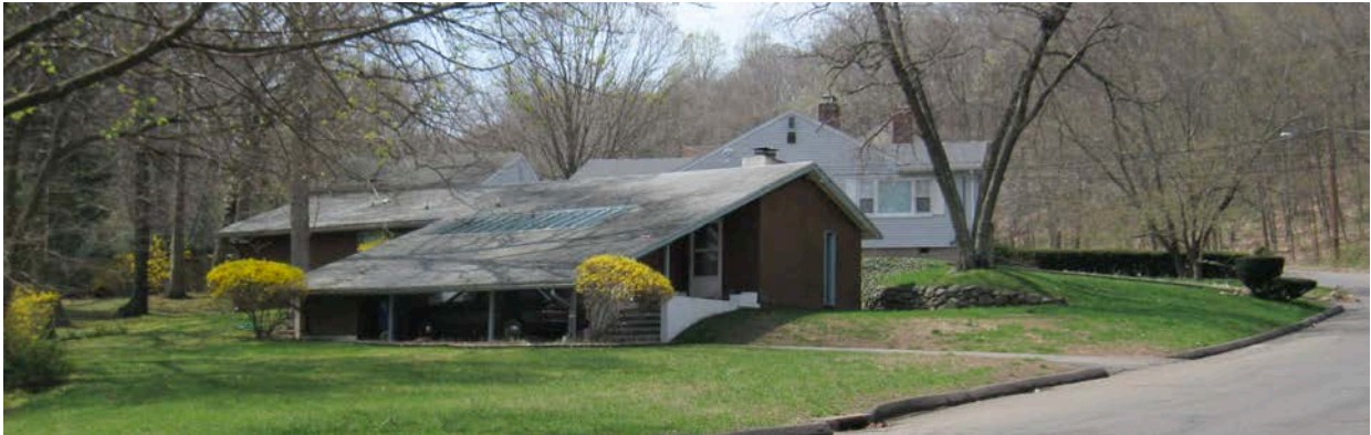
1. Northeast view from Seneca Road, camera facing southwest.
