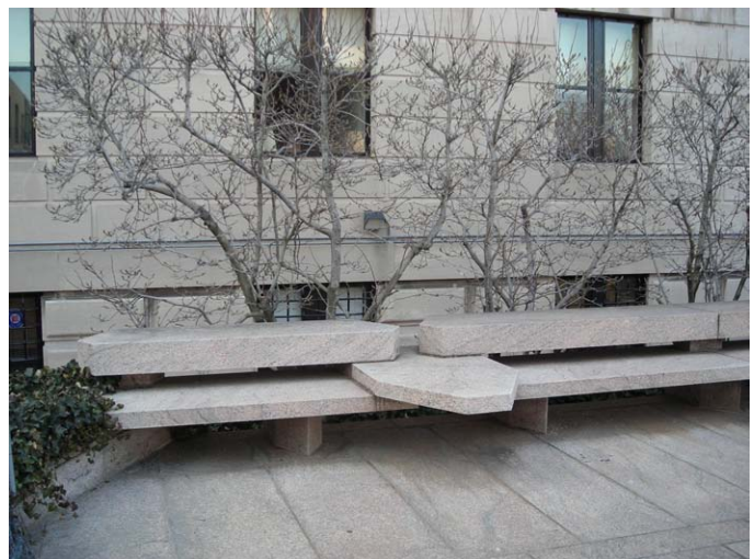
3. Detail view of seating, camera facing west.
