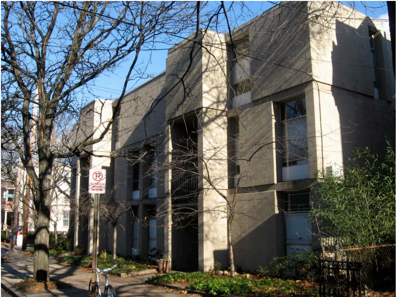
1. Southwest view of 3-story front building from Olive Street, camera facing northeast.
