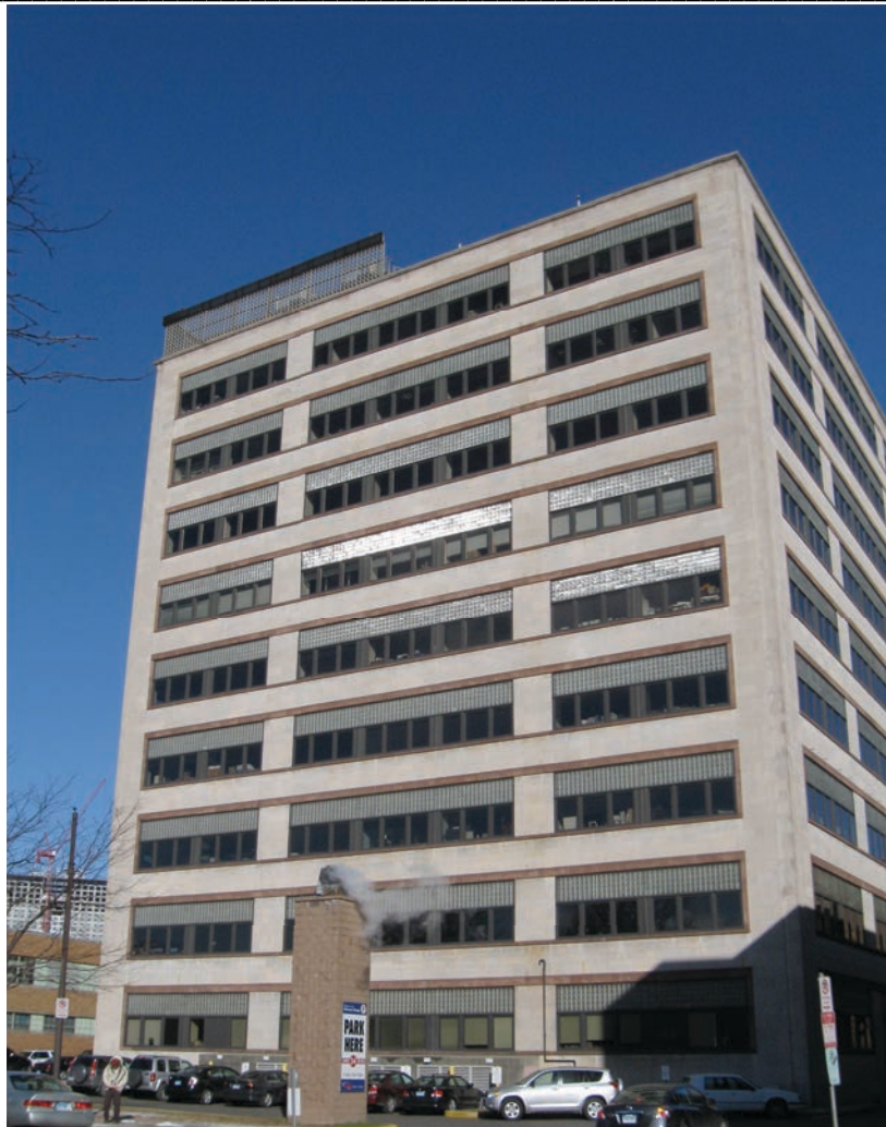
1. Southwest view from street, camera facing northwest.
