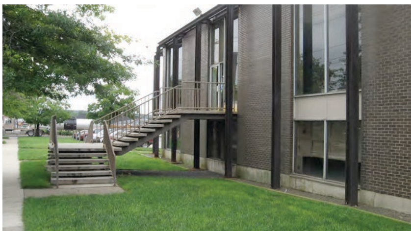
3. Detail view of the building's exterior.
