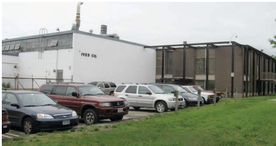
2. North view of the building from the west side.
