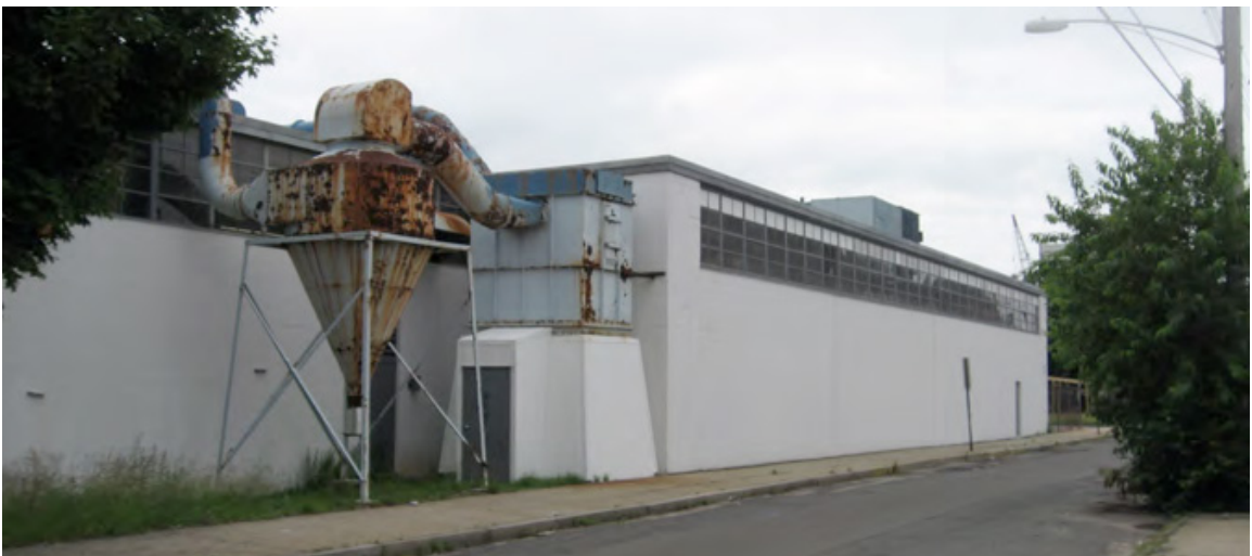
5. West elevation facing Wallace Street, camera facing southeast.
