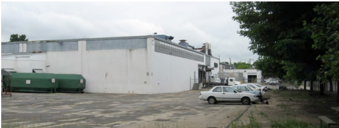
6. Southeast view of rear and East Street elevations, camera facing northwest.
