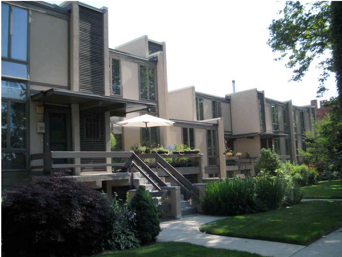
3. South elevation facing Greene Street, camera facing northeast.
