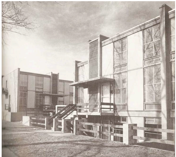
5. Detail, south elevation in 1965, Metz p. 57.
