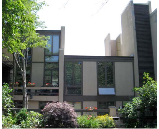
7. West elevation detail, Hughes Place, showing the three-bedroom unit between tall blocks.
