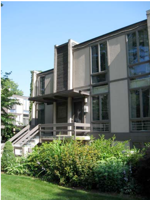
4. Detail of south elevation.
