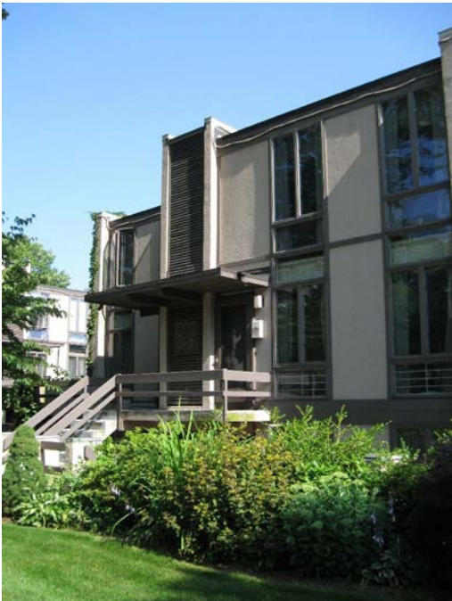
4. a. Detail of south elevation.
