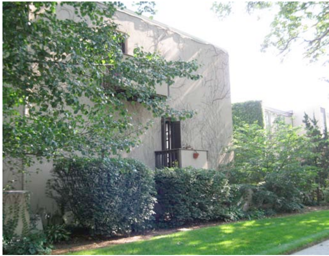
6. South (end) elevation of Hughes Place block.
