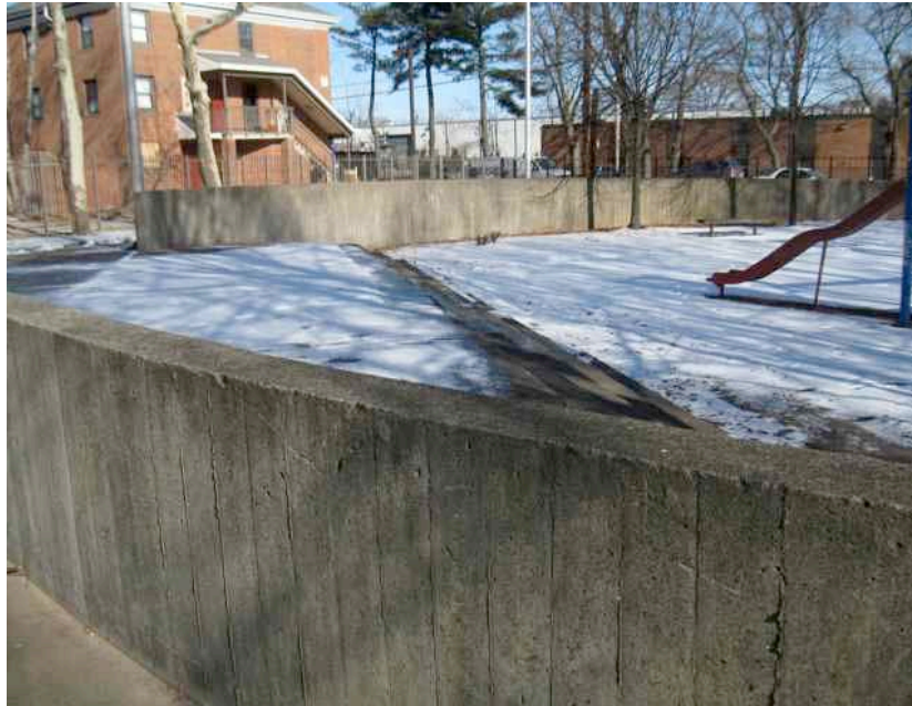
1. View of eastern playground circle, camera facing northeast.
