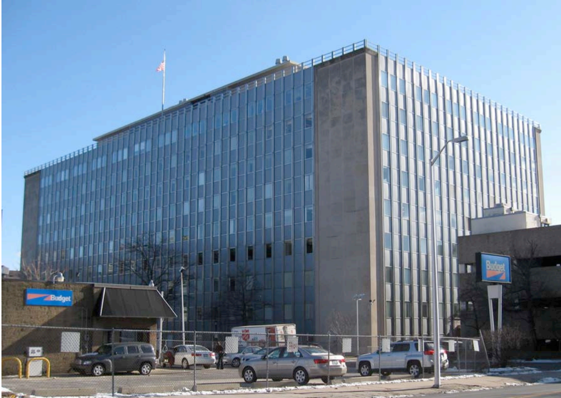
1. Northwest view from High Street, camera facing southeast.
