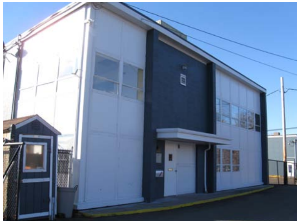
2. North view (front), camera facing southwest.
