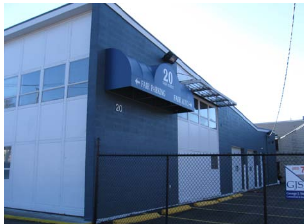
3. West view, camera facing southeast.
