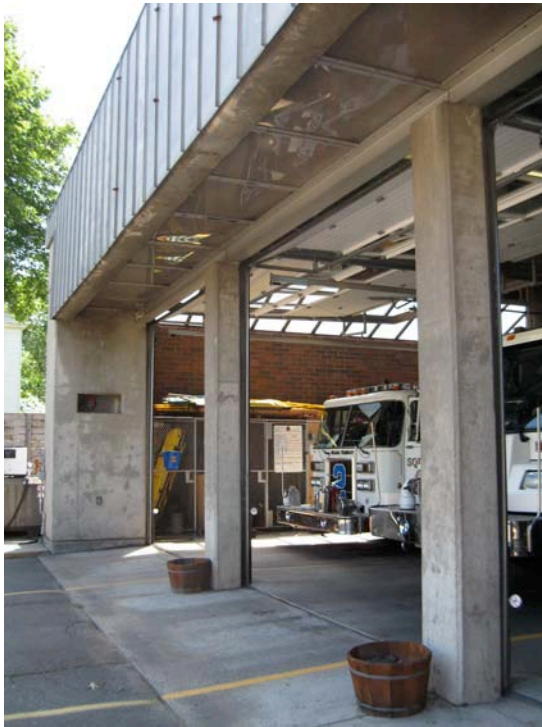
6. East front doors, view of skylights, camera facing south.
