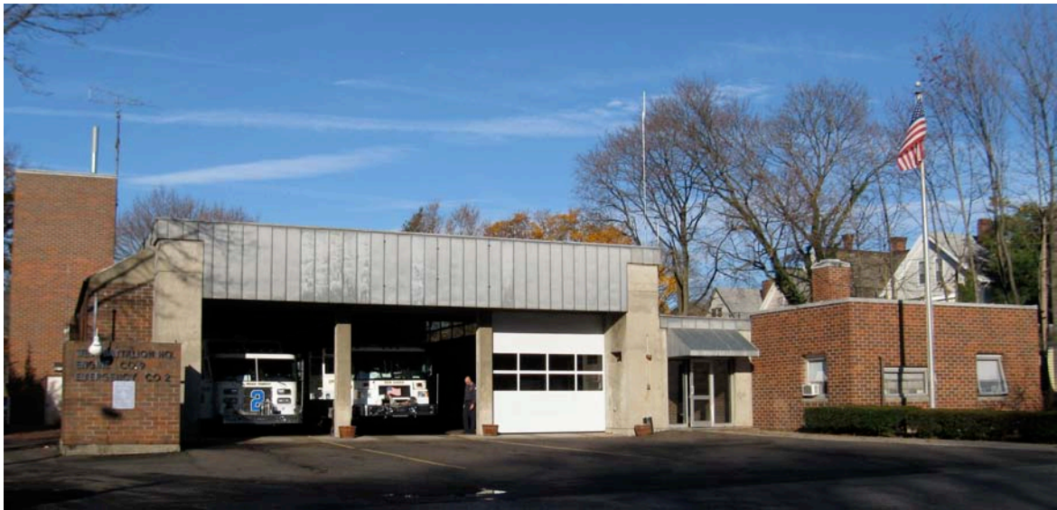
1. East elevation from Ellsworth Avenue, camera facing west.
