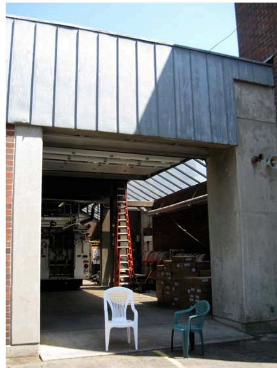
7. West rear door, view of skylights, camera facing southeast.
