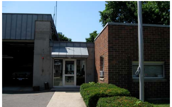
3. East detail of pedestrian entry, camera facing west.
