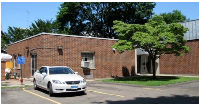
4. Southwest view of rear of building, camera facing north.
