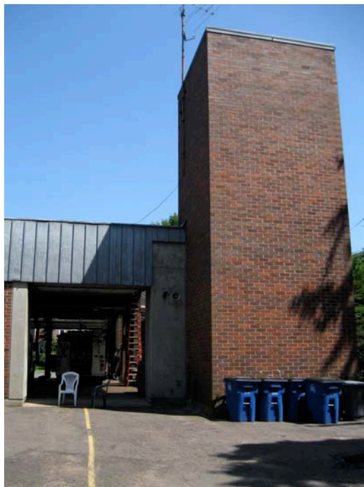
8. West rear view of hose tower, camera facing east.
