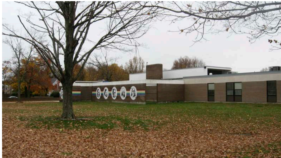
3. East (front) and north (side) elevations from Dixwell Avenue, camera facing southwest.
