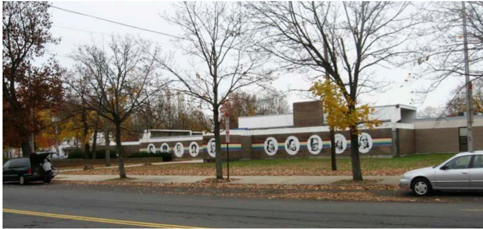
2. East (front) elevation from Dixwell Avenue, camera facing southwest.
