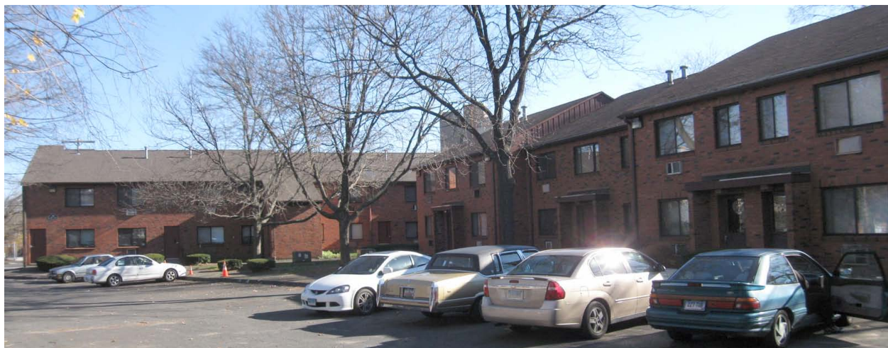
2. Northwest view, camera facing east. Rear of east building at left; north front of west building at right.
