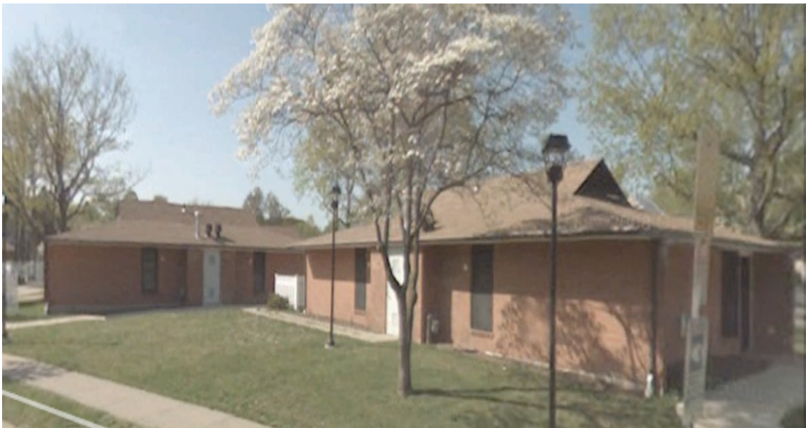
View from corner of Daisy and Goodyear, camera facing southeast.
