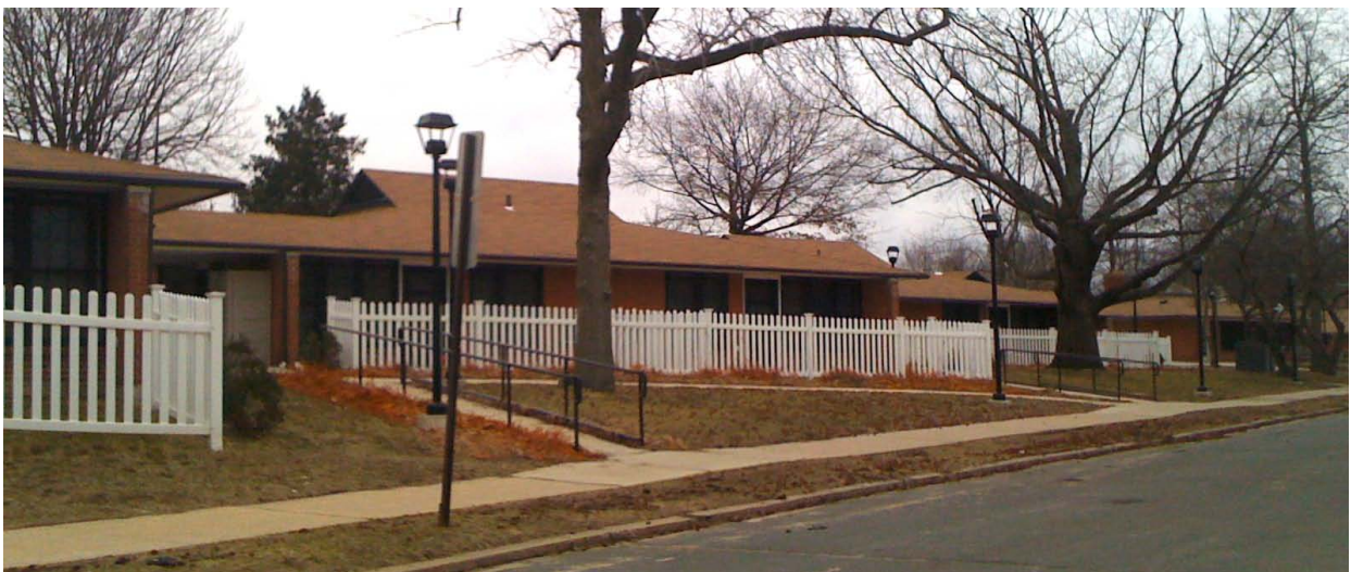
1. South view from Daisy Street, camera facing northeast.
