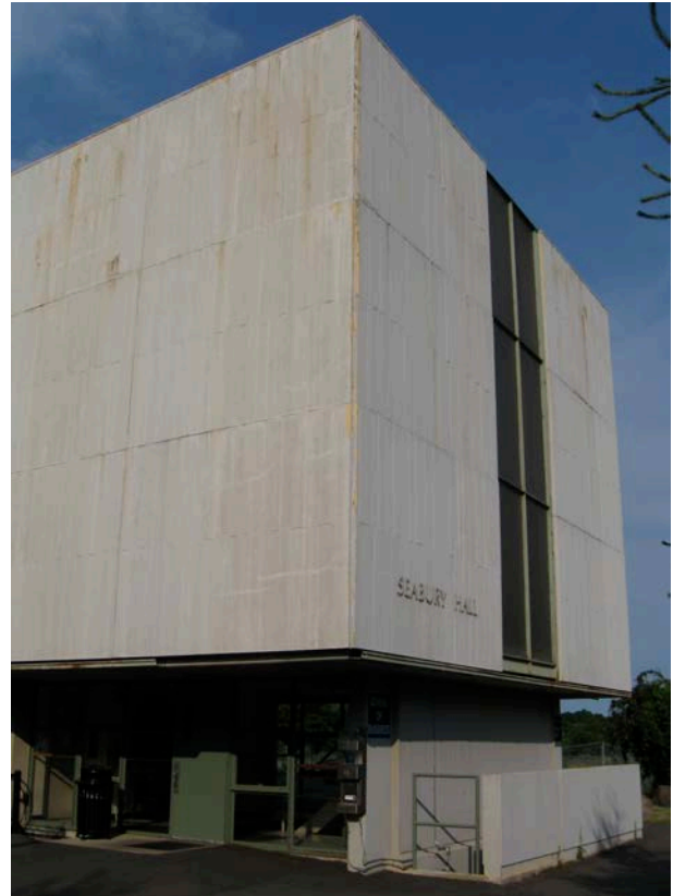
4. Southwest view, camera facing northeast.
