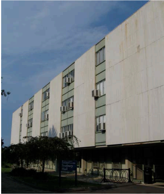
3. West view, camera facing northeast.
