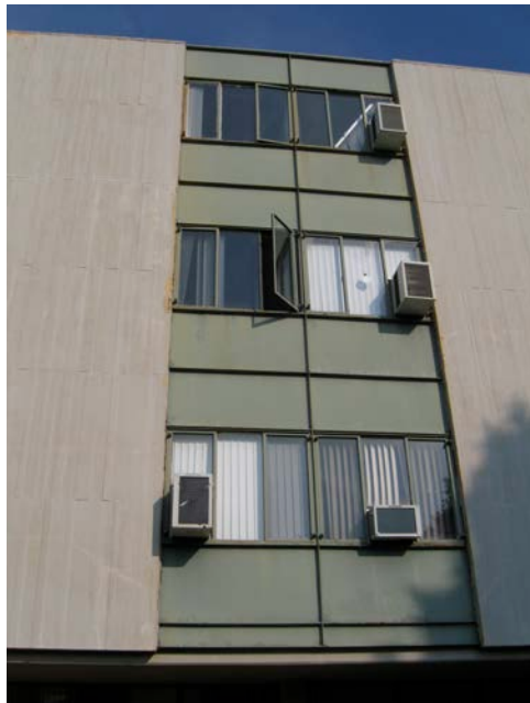
5. Detail of curtain wall with windows, camera facing east.
