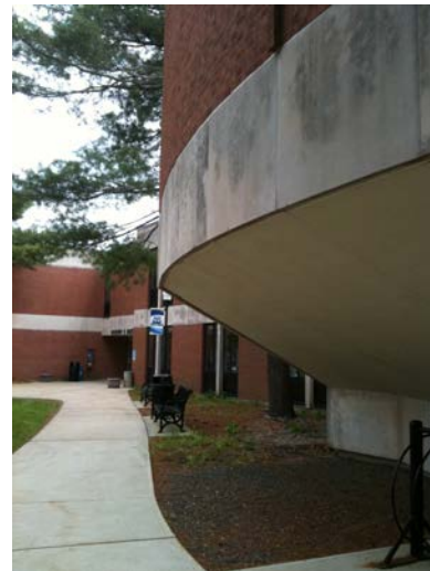
4. View of cantilevered lecture hall and building main entrance, camera facing east.
