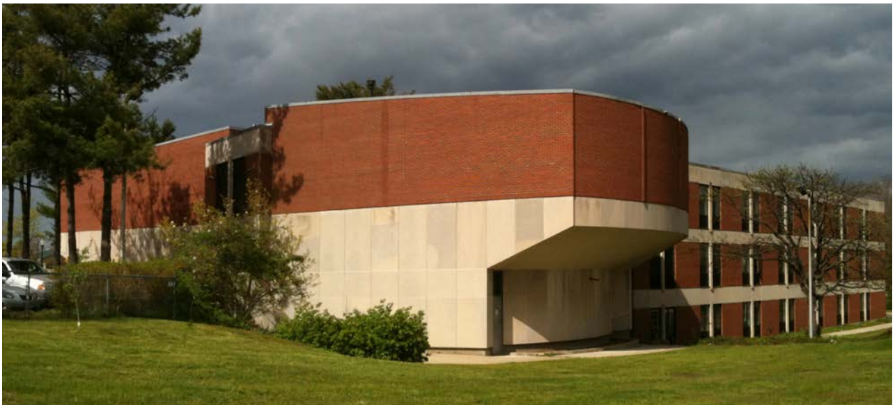
1. Southwest view of lecture hall wing, camera facing north.
