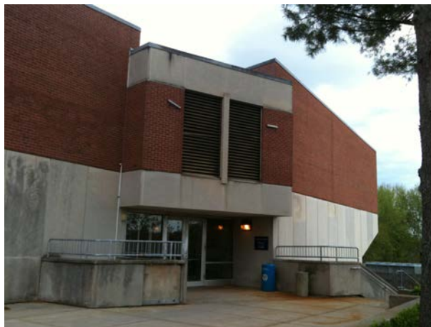
3. West exit plaza from lecture hall wing, note mechanical louvers used as sculptural form; note missing limestone slab, illustrating use of limestone for similar effect to raw concrete, camera facing east.
