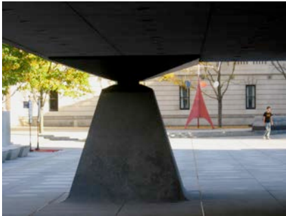
Tapered pedestal, Beinecke Rare Book and Manuscript Library (1960–63), Skidmore, Owings and Merrill, architects. Photo looking east. A stabile by Alexander Calder stands in the plaza.
