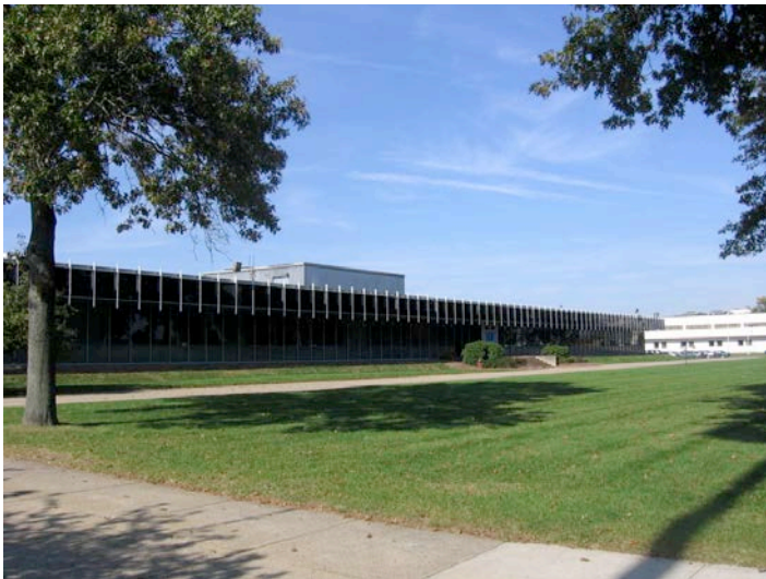
Sargent and Company Headquarters (1964–66), Orr, deCossy Winder and Associates and Pederson & Tilney, architects. Photo looking northwest.
