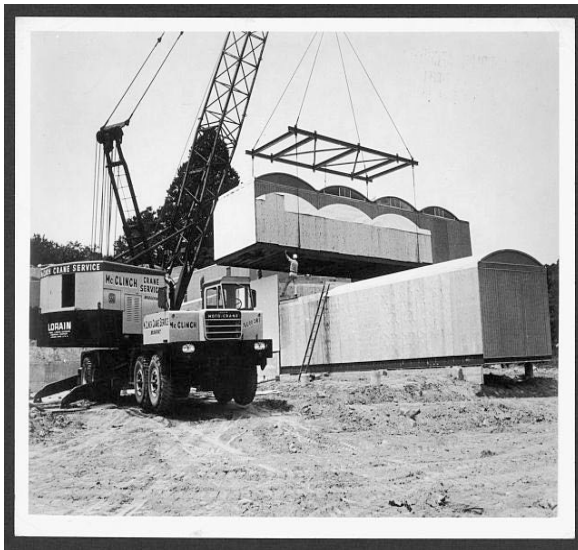
Old-fashioned box raising at Oriental Masonic Gardens, 1968, Paul Rudolph, architect. Courtesy of the Prints and Photographs Division, Library of Congress.
